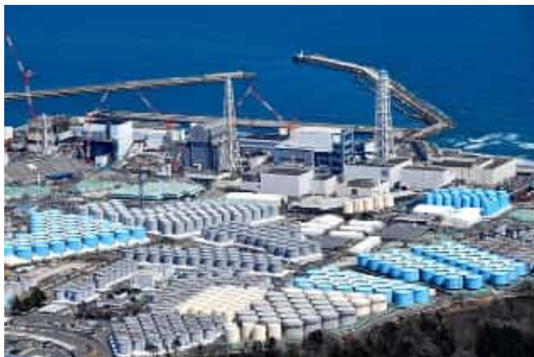
Tank farm at Fukushima, from which radioactive water is being released into the Pacific Ocean. Photo, The Asahi Shimbun, Nov. 7, 2022. https://www.asahi.com/ajw/articles/14762193
